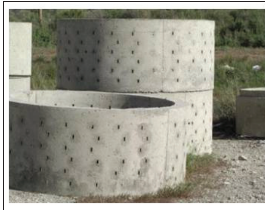
Figure E.4. Dry Well #1 – Structural Prefabricated Chamber.
